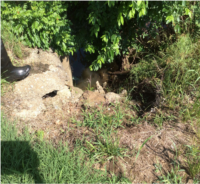
PHOTO 1 Description Erosion behind the Northeast wing wall.
