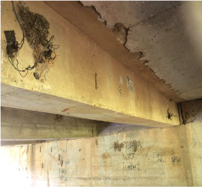
PHOTO 1 Description Girder # 3 spalling with exposed reinforcing steel.
